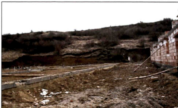
Fig. 6.5 Active part of landslide - undercutting of landslide toe (photo: Kopecký, 2008, in Trangoš, 2013)
